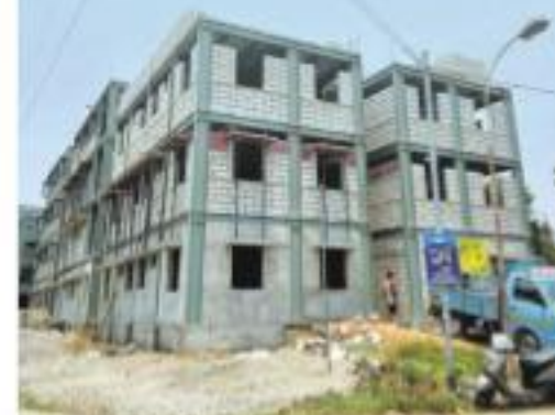
room, daycare centre, administration room, reading room, rainwater harvesting system, potable water system and fire-fighting system.
